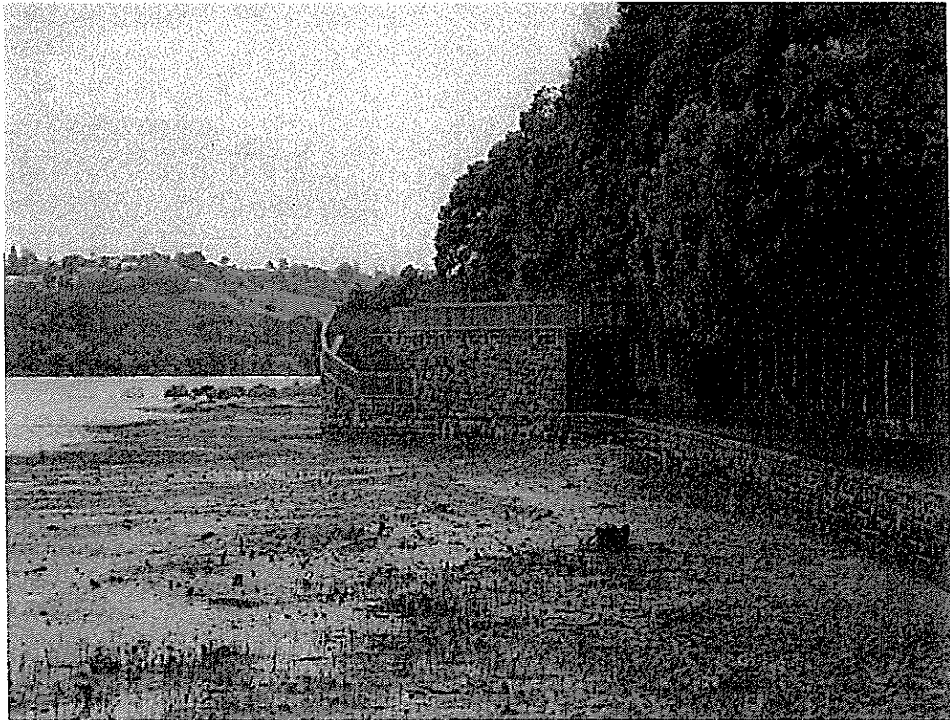
Victoria Ave Drop Shaft - 14/07/11
